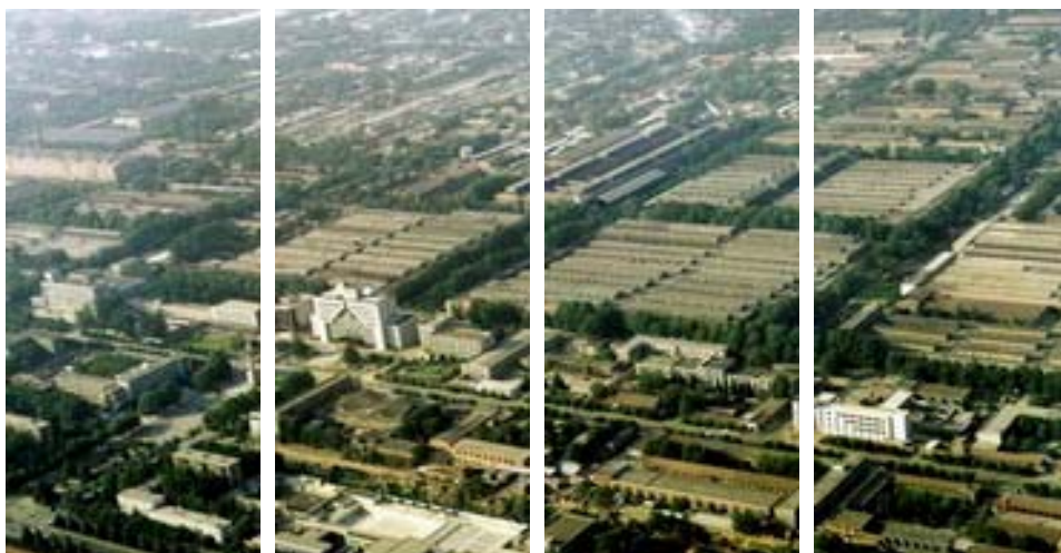
Aerial view of the LYC facility in Luoyang
